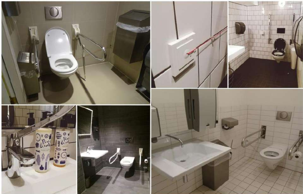
Image 13: Example of lever type tap, foldable grab bars, etc. in accessible toilet type A (Source: https://www.ableamsterdam.com/wp-content/uploads/2019/06/accessible-toilets-2-1024x662.jpg )
