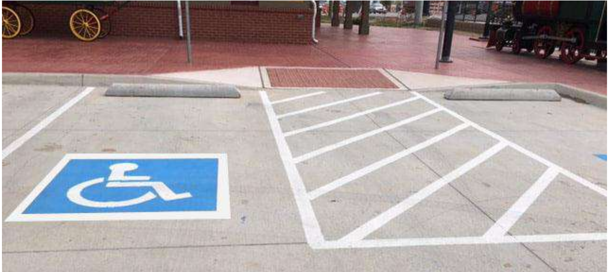
Image 1: Example of parking symbol on floor, transfer bay marking and kerb ramp
