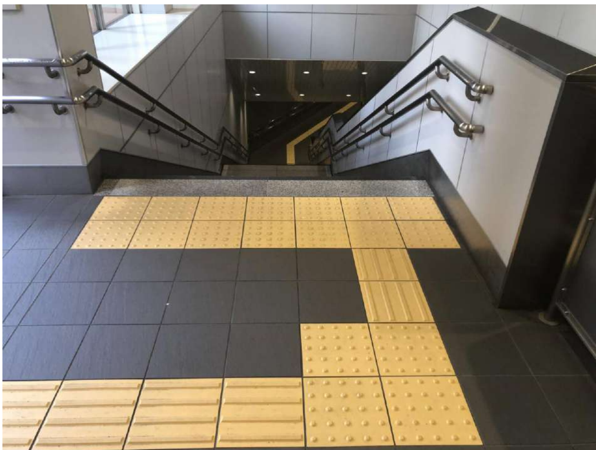
Image 10: Example of tactile flooring provided at the beginning of the staircase and handrails at two levels (Source: https://cdn-japantimes.com/wp-content/uploads/2020/08/np_file_30691.jpeg )
